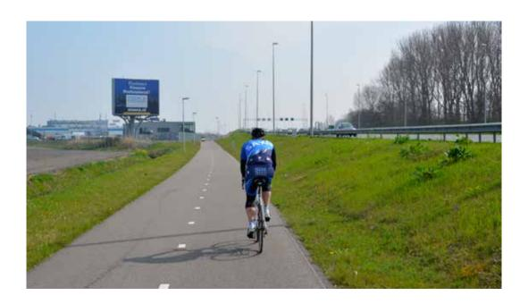
Cycle tracks along major roads must always be fully segregated with a distance of between 4 and 8 metres from the main carriageway. This provides sufficient overlooking from cars to provide visual safety whilst also being far enough away to reduce the noise of the traffic. Ideally trees should be planted in this space.
