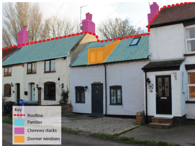
Figure 22 Roof features and materials in Lound
