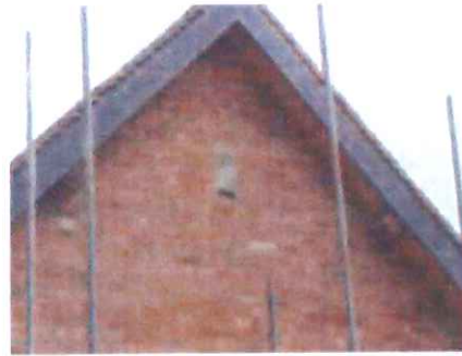
Fig. 24 Schweger 1 FR bat tube Fig. 25 Bat tube installed in gable end
