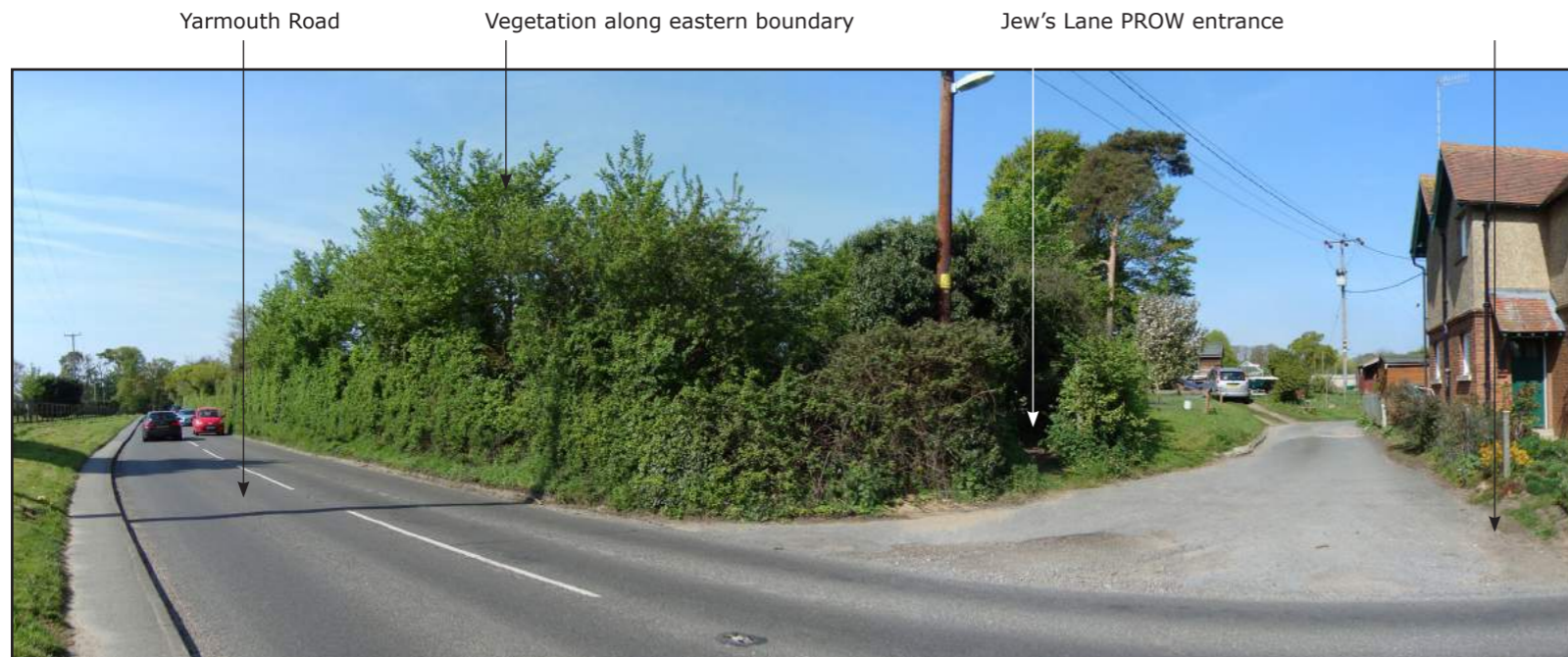
Photograph 1a - View south along Yarmouth Road opposite site
