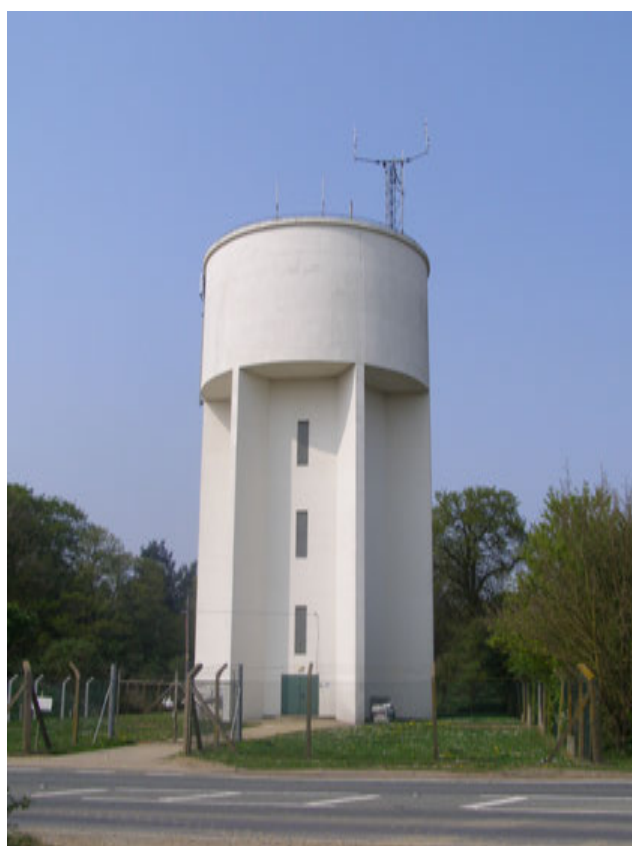
The water tower, A1152
