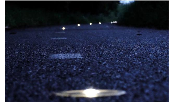
**Figure 23:** Example of a foot/cycle path which is lit by solar cat's-eye providing some light for pedestrian and cyclists without creating any disturbance to the nearby properties or unacceptable levels of light pollution.
