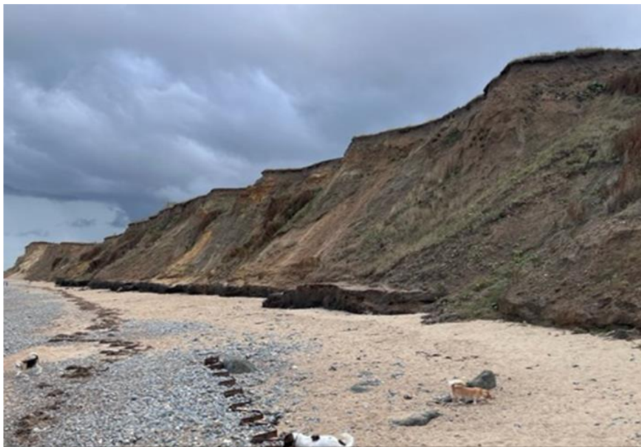
Eroded cliffs at East Runton showing old sea defences.
