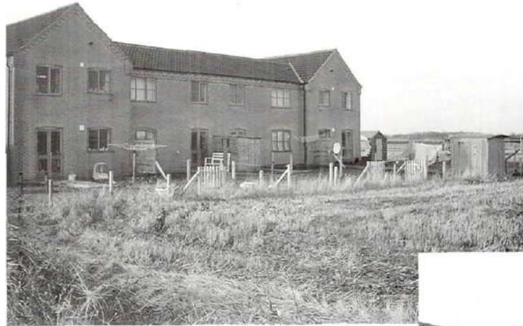
Unscreened rear gardens.
