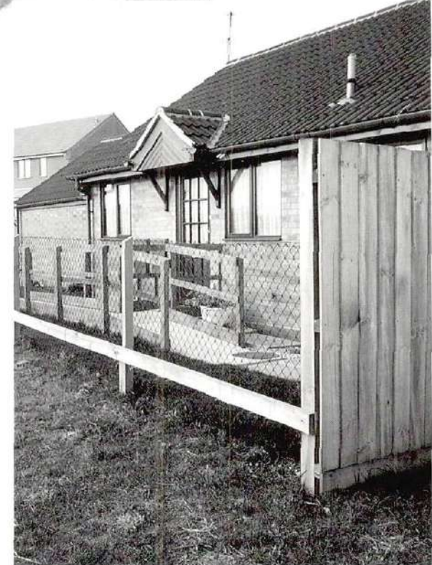
Fencing which detracts from the appearance of property.
