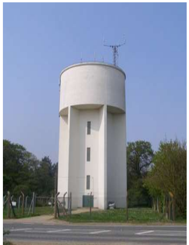
The water tower, A1152
