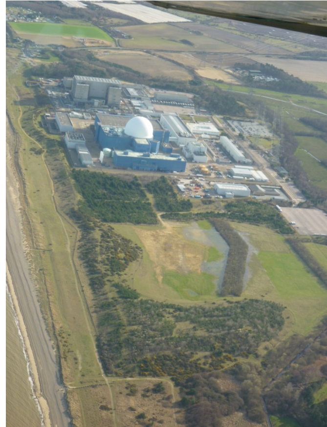
Sizewell A, Sizewell B and the Sizewell C site to the north
