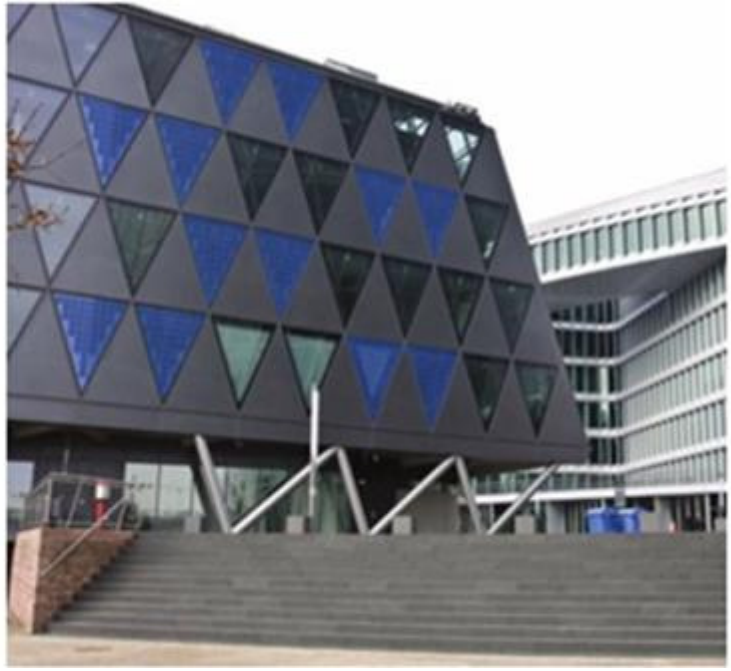
Figure 2. Flat Panel system metal cladding / rain screen cladding
