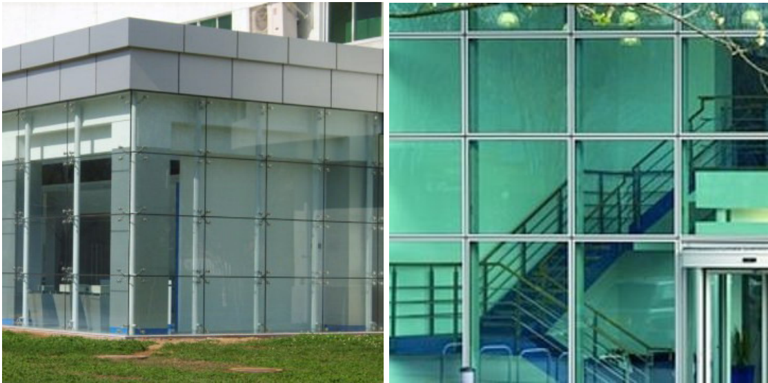
Figure 6. Framed and Frameless Glass Curtain Walls
