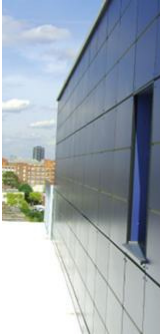
Figure 2. Flat Panel system metal cladding / rain screen cladding
