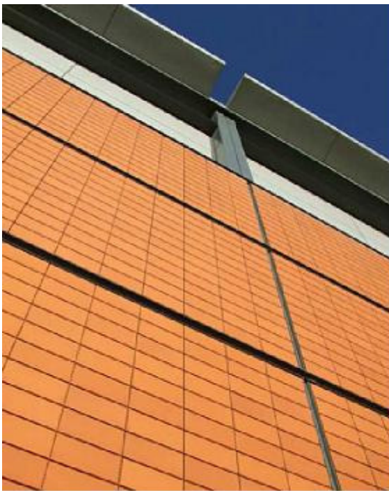
Figure 3. Terracotta rain screen cladding
