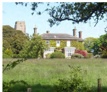
Property at risk of erosion in Covehithe
