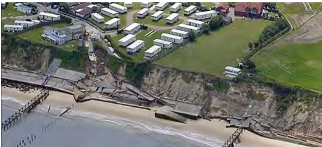
Aerial view of Corton seawall collapse
