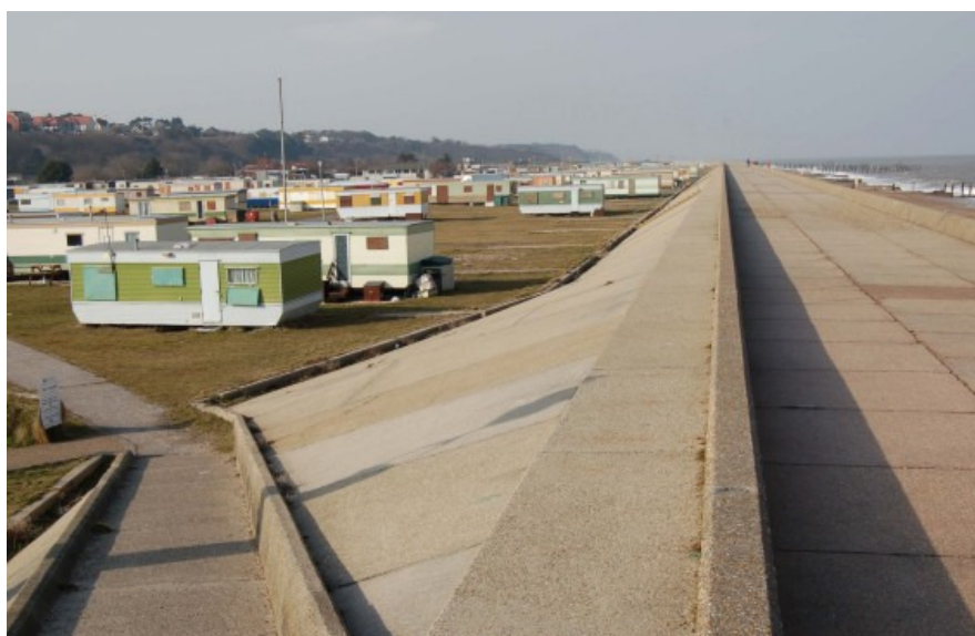
View of Area C looking from the southeast sea wall
