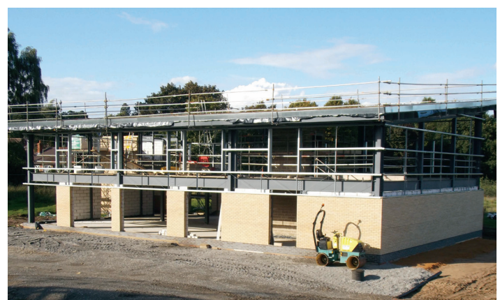
Work is progressing well
