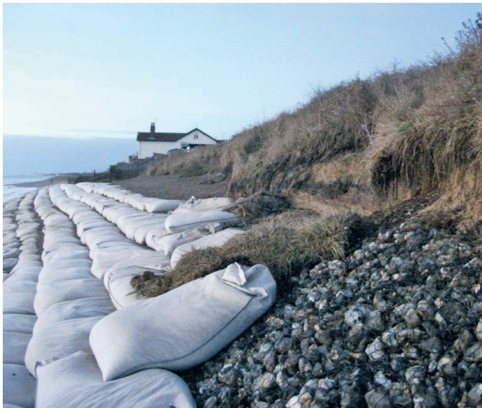
Flooding in December 2013
