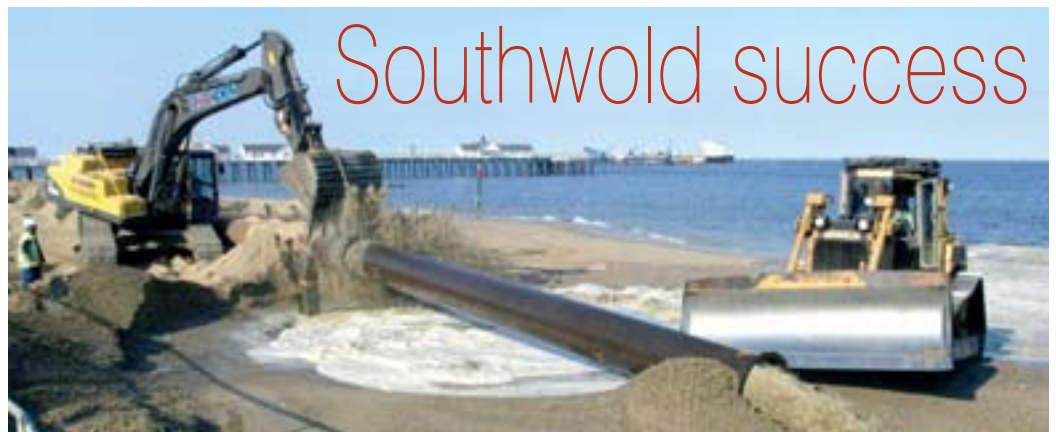
Work continues apace on Southwold beach
