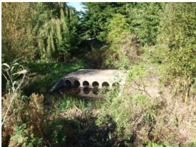
Piped inlet into the flood storage area (after clearance)
